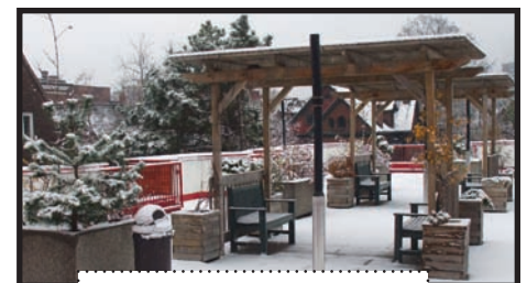
First snowfall of the season on the Terrace rooftop garden.
