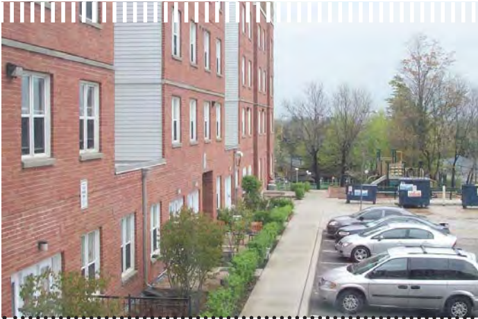
Sewells Road parking and ground-floor patios.
